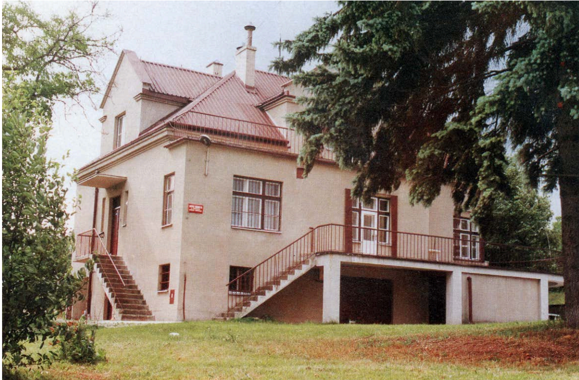
Field Station of the Department of Ecology in Szarów
